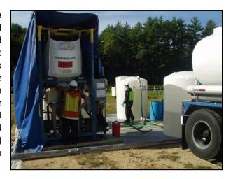
Treatment in Area A was focused on parcels A-11, A-14 and A-15. A total of 7,350 gallons of hydrogen peroxide were injected into 13 wells (Phase II), 25,800 gallons of ALK-ASP were injected into 35 wells (Phase III), and 22,990 gallons of MFR were injected into 34 wells (Phase III).
