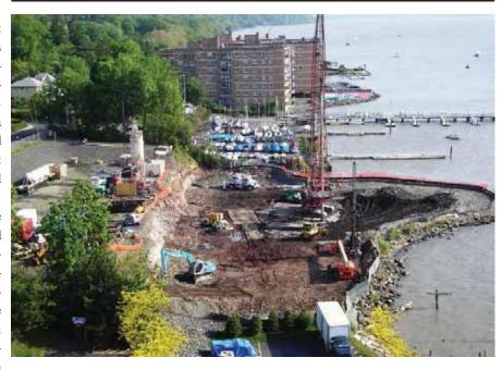
vided the site into upper and lower terraces to provide sufficient staging room for the remainder of the remediation process. Approximately 36,000 tons of contaminated soil were removed and disposed of at an off-site low-temperature thermal desorption facility. Also removed were concrete and brick subsurface foundations leftover from the gas plant's demolished structures and storage tanks, and timbers from decayed waterfront structures.
